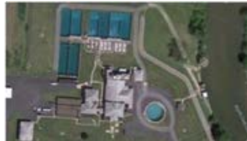
Figure 11: Newark Water Treatment Plant
